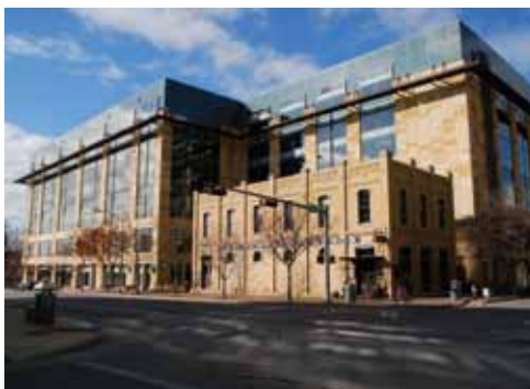
The former J. P. Schneider store, 1873, and one of the Computer Sciences Corporation headquarters buildings, 2001, Austin, TX
